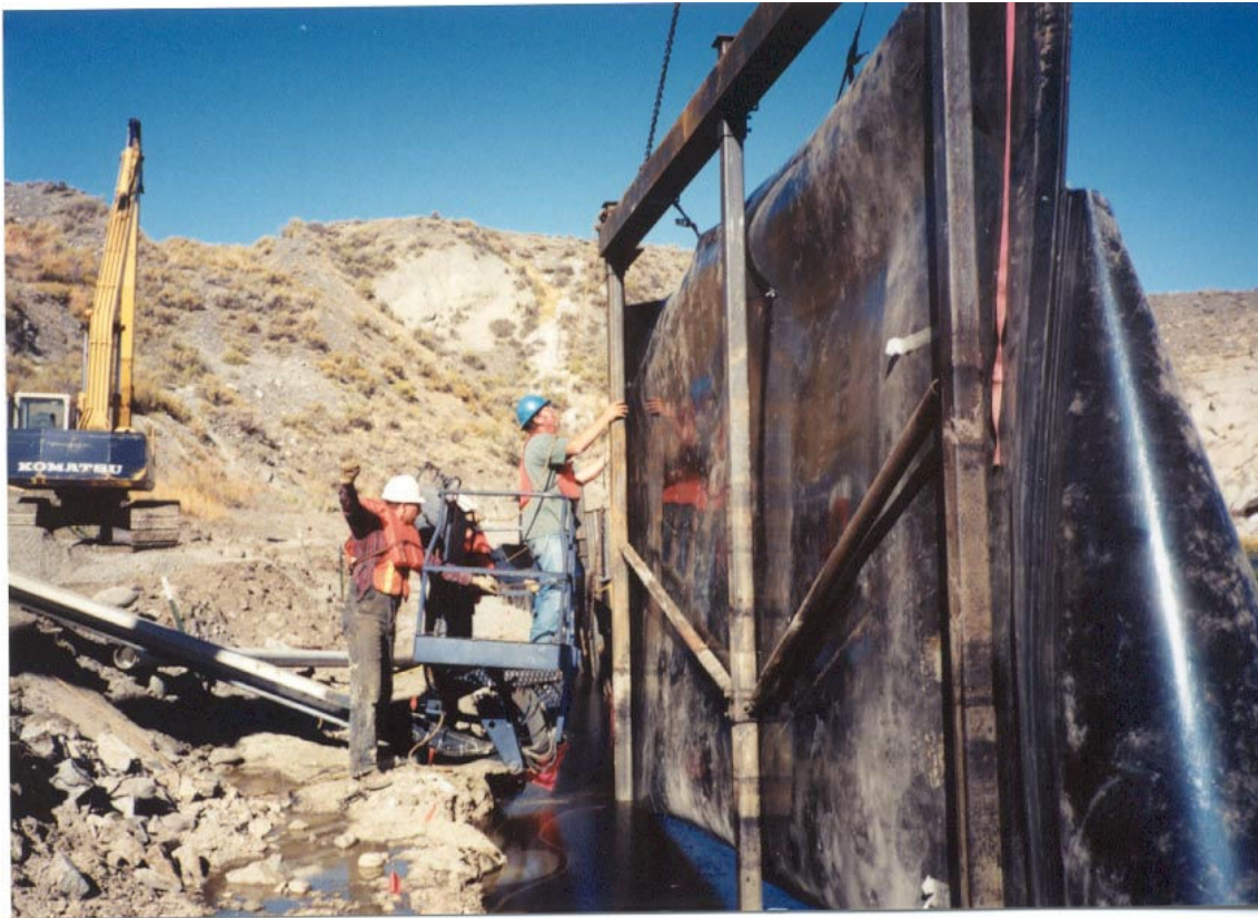
Figure 3. Installation of liner in slurry wall using temporary steel frame
