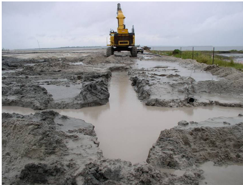
Figure 5. Excavating the trench supported by bentonite slurry
