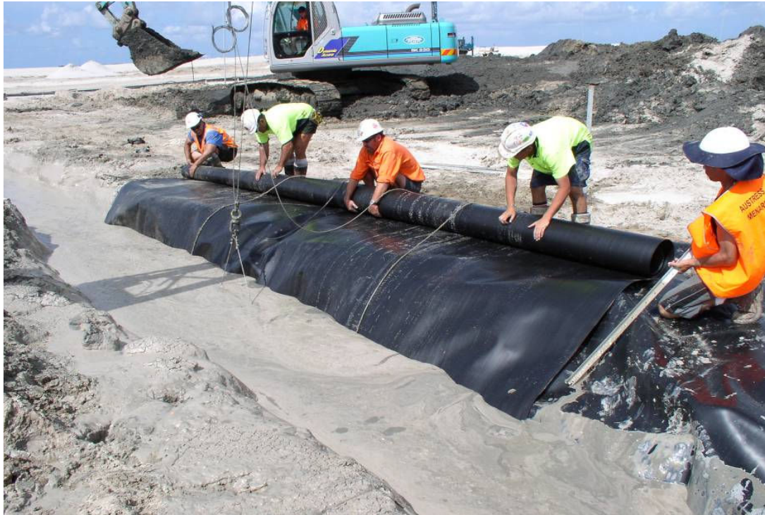
Figure 6. Placing HDPE panels vertically with overlap
