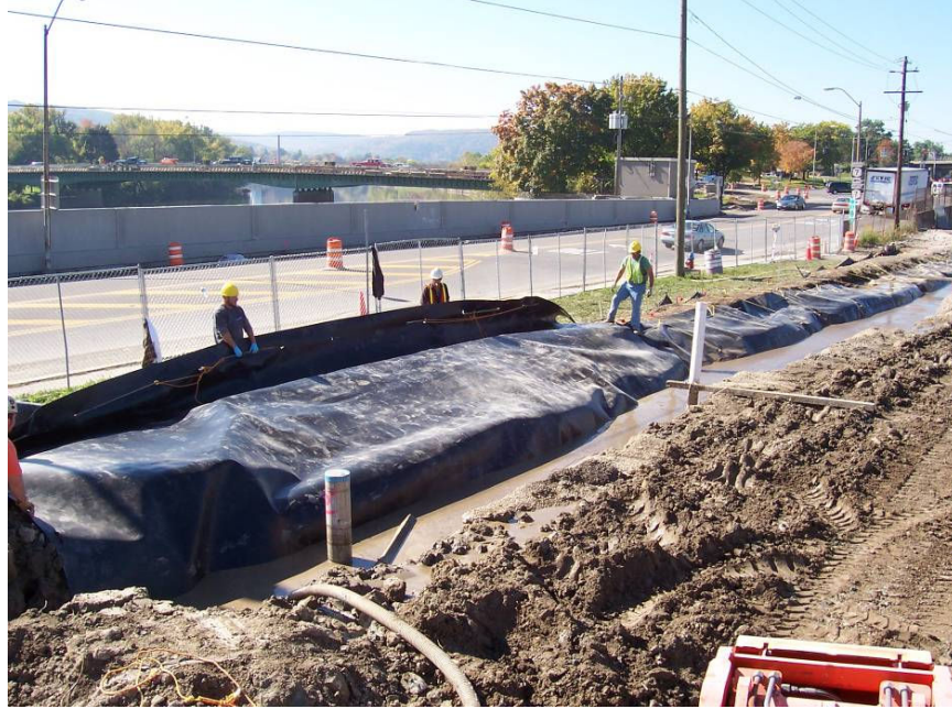
Figure 4. Liner being placed with overlapped joints
