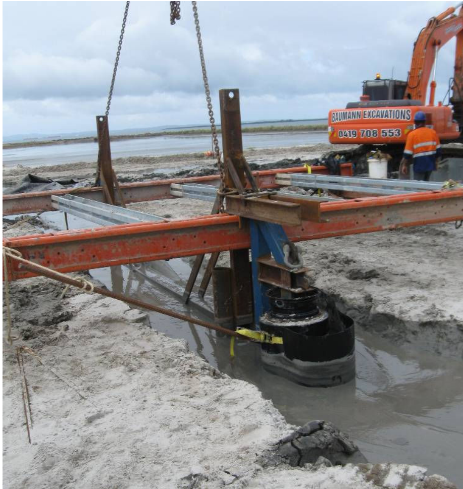
Figure 7. Placing the HDPE liner with a horizontal roller.
