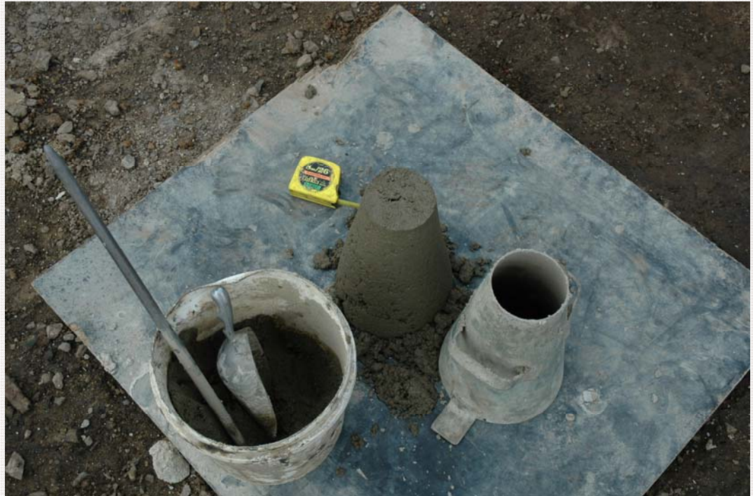
Typical low-slump test outcome for compaction grout
